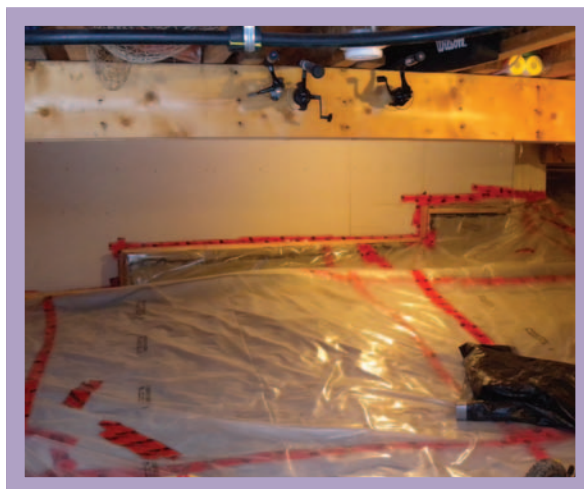
Photo 6 – Membrane and Wall Attachment
