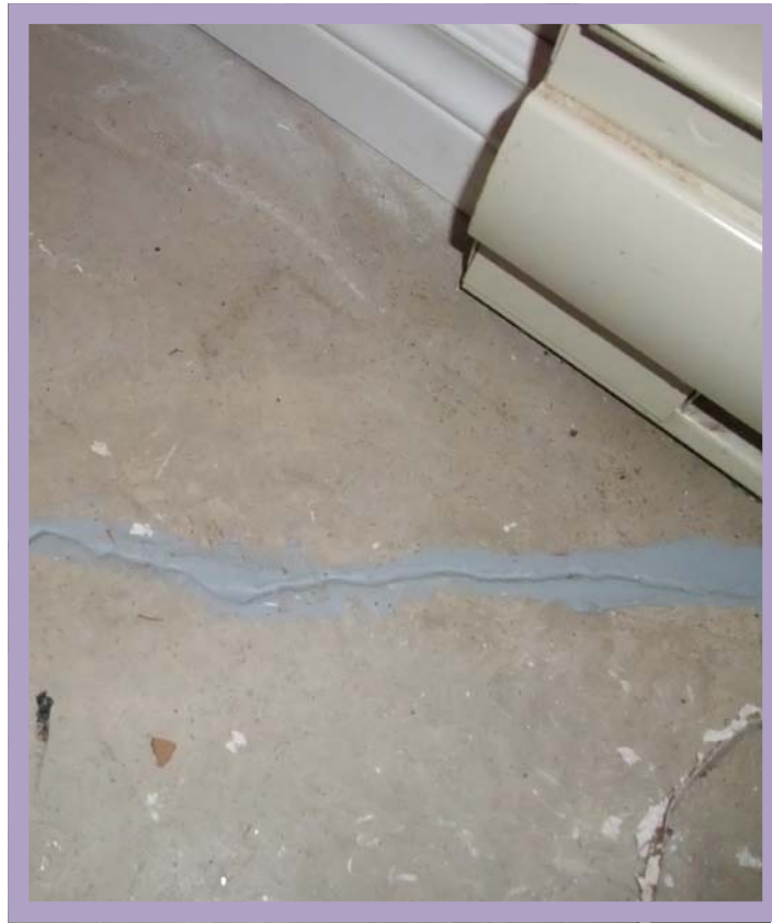
Photo 8 – Sealed Crack in Concrete Slab
